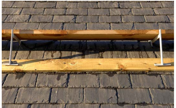
Photo 3. A typical roof on completion. Before removal of heels
