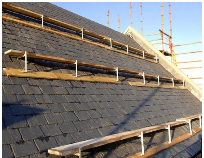
Photo 3. A typical roof on completion. Before removal of heels
