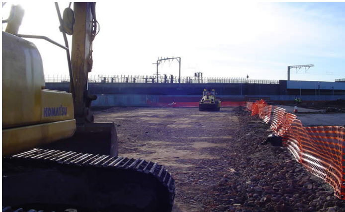
Construction of a Piling Platform
