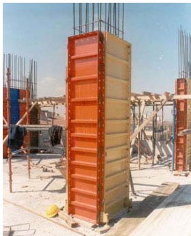
Formwork (Shuttering)
