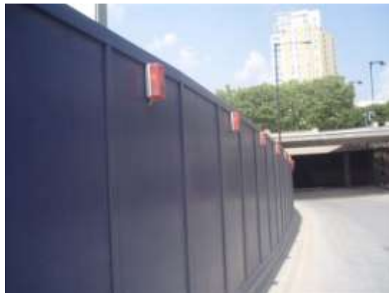
Site perimeter hoarding
