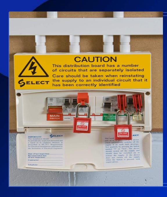
Example of use of circuitbreaker lockouts
