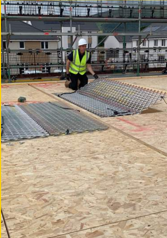
Stairwell Void Fully Protected
