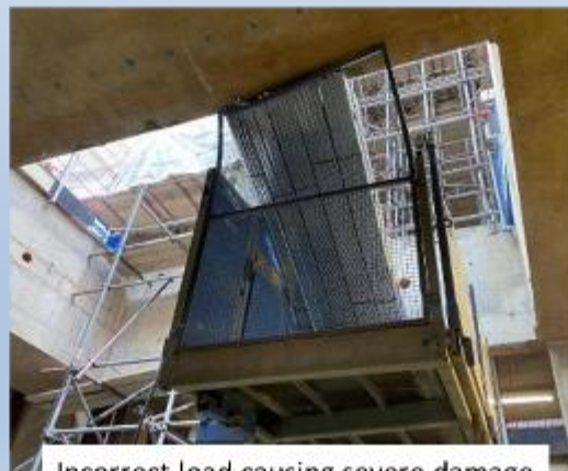
Incorrect load causing severe damage
