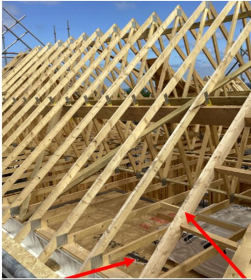
Open truss system with progressive install of wrap a round system working up the roof
