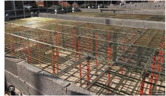
Safety decks underneath trusses
