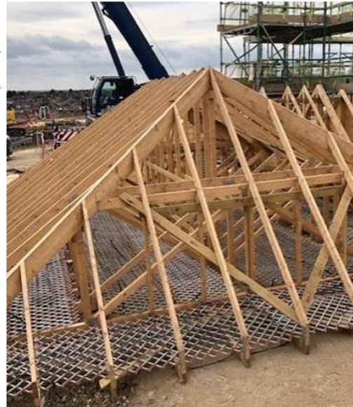
Trellis decking installed into trusses
