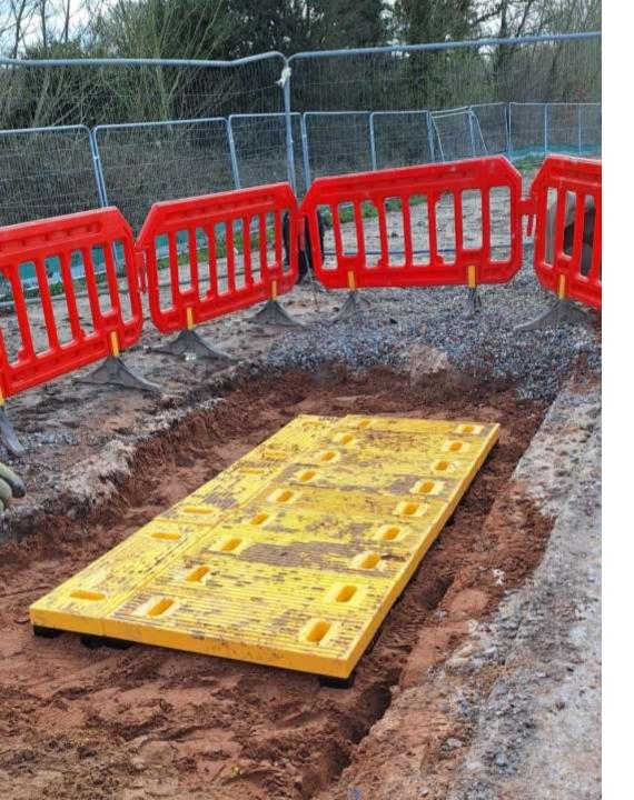
Strike Matz is a new Utility Protection System to prevent Cable Strikes whilst Excavating to expose Underground Services.
