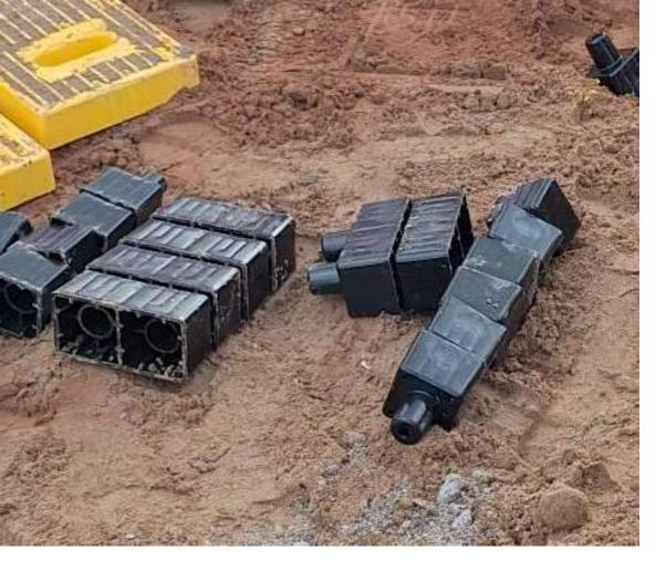
Packs can be configured rectangular to provide Plot Connection protection, or in a continuous run over a service, length or width ways, depending on the diameter of the Services.
