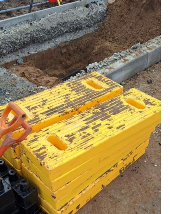
Boards are constructed from specialist High-Density Polyethylene to allow for maximum impact resistance.
