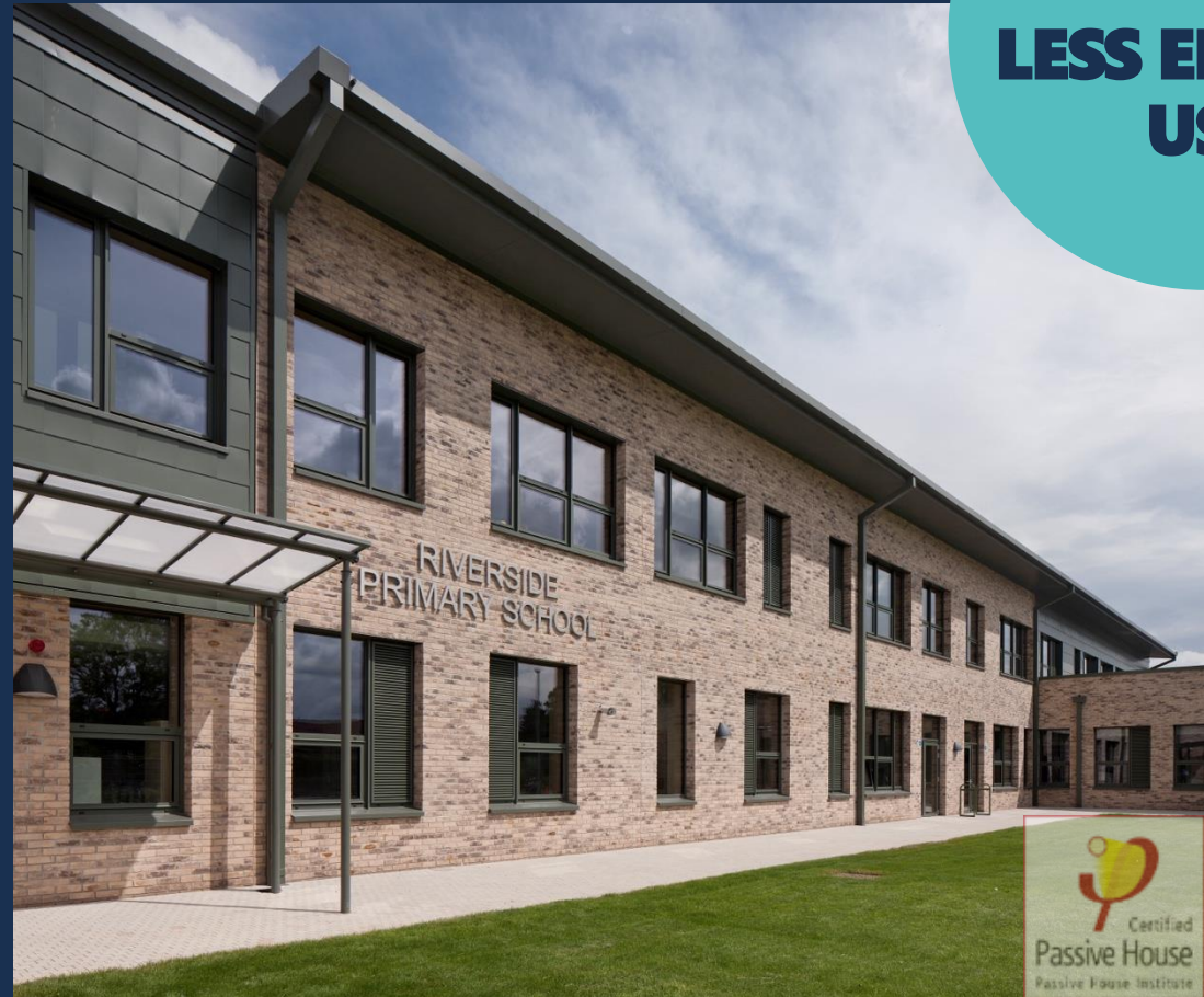
Riverside PS, Robertson Construction
