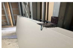
Site solution using bracket/ bolt
